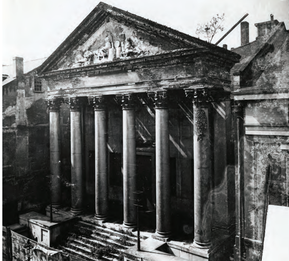
The former Citizen’s Bank (1838) on 620 Toulouse St. looked like a Greek ruin in its last years. This scene dates to around 1898, ten years prior to the building’s demolition. Courtesy Library of Congress
